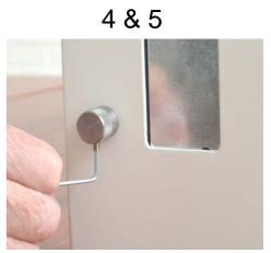
Striking plate: adjustable position by using the 2 screws
