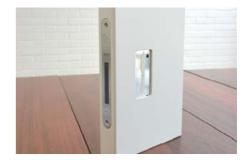
After testing the lock install the finished coverplates.
